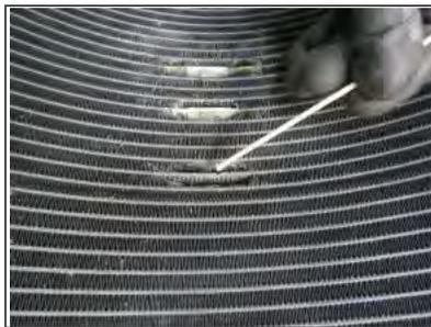
14. The vacuum pump should be able to pull the epoxy through the cut area to form a shape that works as a plug.
