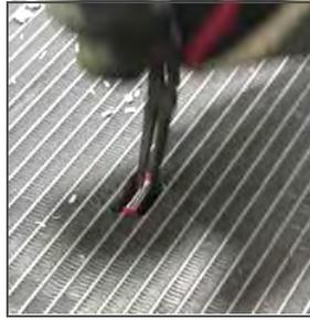
18. Allow an additional one to two hours for epoxy to cure before leak checking the system.
