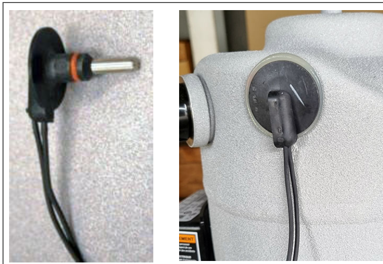
Figure 7.25 Compressor Discharge Temperature Sensor (CPDS)
