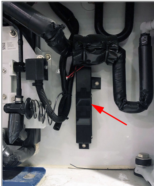
Figure 3.29 Supply Temperature Sensor (STS) / Supply Recorder Sensor (SRS)
