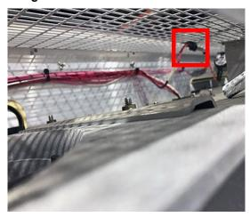
Figure 7.20 Return Sensors - Bracket
