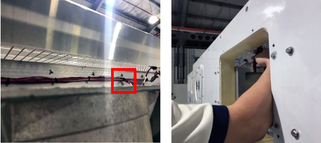
Figure 7.29 Return Sensors - Cutting Wire Ties
