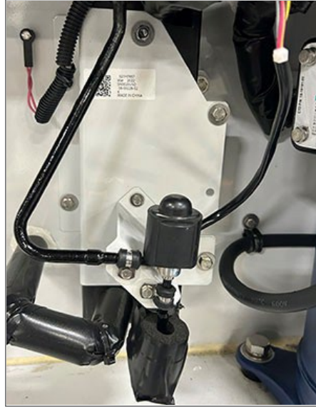
Abbildung 7.17 Economizer-Expansionsventil (ECV)
