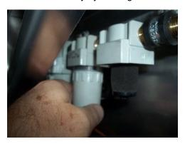
8. Lubricate the O-ring on the first filter housing and reinstall onto the filter body by rotating clockwise into the base.
