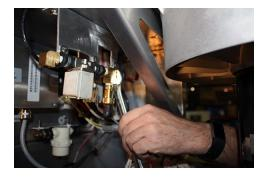
5. Remove the three 1/4" x 20 screws with a 7/16" socket and remove the coil assembly.
