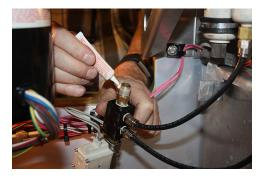
12. Reconnect the VPS apply cable tie and refit the access panel.
