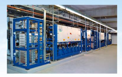
Latest generation of  $\mathrm{CO}_2$  transcritical systems,  $\mathrm{CO}_2\mathrm{OLtecEvo}^{\otimes}$  provides energy efficient and environmentally sustainable refrigeration, through our patented modulating ejector technology and a  $\mathrm{CO}_2$  pump.
