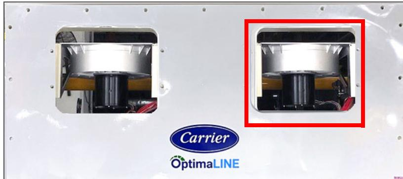
3. Loosen the fastener on the sensor bracket.
