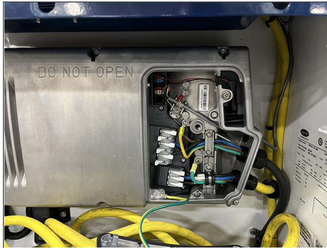
4. Release both sets of wires (compressor power cable and line power cable) from the VFD terminals. Make a note of the exact wire position as the same connections must be done on the replacement VFD.
