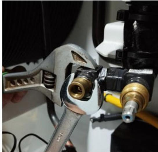
3. Unscrew the cap for the high side charge port at the discharge service valve.
