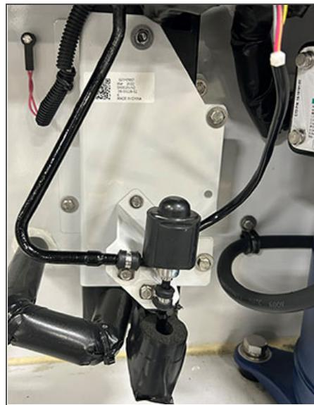
The Electronic Expansion Valve (EEV), as shown in [Figure 7.18](#), maintains superheat of the refrigerant gas leaving the evaporator. The valve functions are: (a) automatic response of refrigerant flow to match the evaporator load and (b) prevention of liquid refrigerant entering the compressor.
