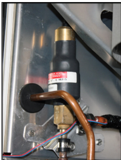
Figure 6 Electronic Expansion Valve (EEV)
