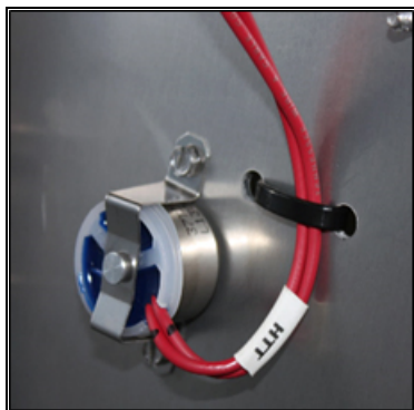
Figure 9 Heater Termination Thermostat (HTT)
