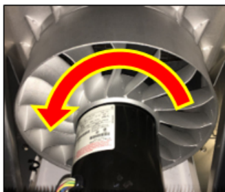
Figure 24 Evaporator Fan Rotation
