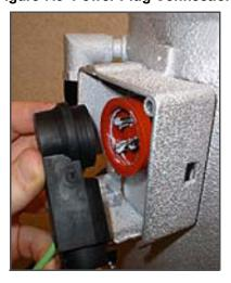
Figure 7.10 Power Plug Secured
